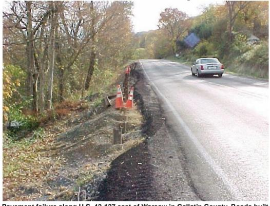
Pavement failure along U.S. 42-127 east of Warsaw in Gallatin County. Roads built on shale slopes can require continued maintenance. The Ohio River is below to the left. Photo by Warren Anderson, Kentucky Geological Survey.
